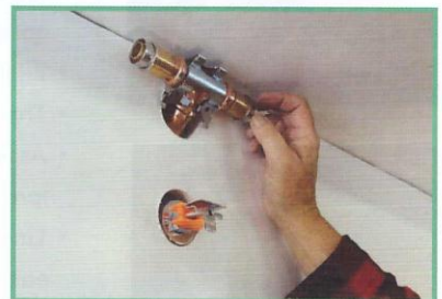
Insert the J-Fit assembly with the attached sprinkler
