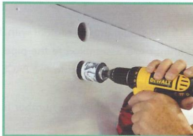
Use a hole saw to cut two holes
