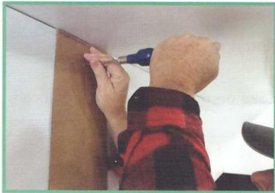
Using the template mark the hole locations
