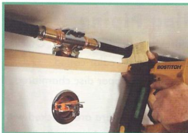
Install the crown moulding
