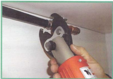
Make the Viega PEX connection
