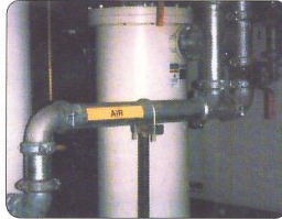
Reverse osmosis grooved end caps allow easy filter membrane service
